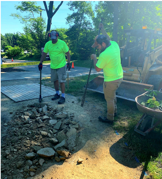
Path construction at Pondview Park
