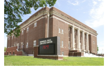
Recently Renovated Memorial Hall Civic Center
