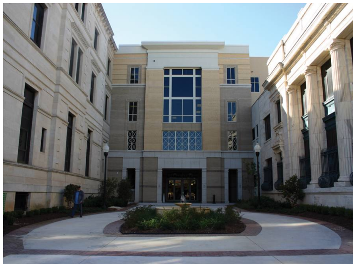
New County Administration Building
