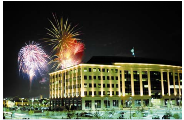
Aurora Municipal Center completed in 2003 houses the City's administrative offices
